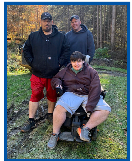
Pictured left to right: Standing Dennis Bashline, Jim Kallenborn from Pine Valley Landscaping; and seated: Alden Bashline, a student at Fretz Middle School. Alden and his family had a gravel pathway installed from their home to their driveway to make the trip to the school bus more accessible.
